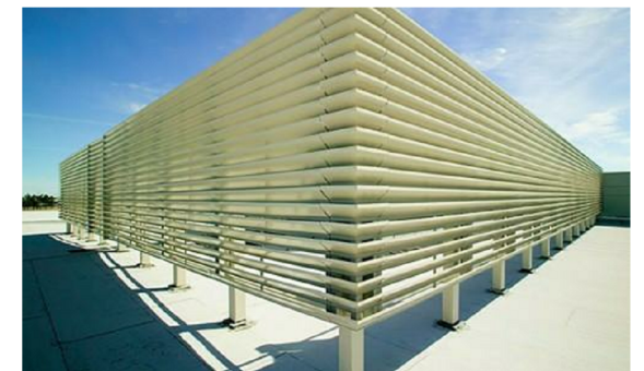
5. PENTHOUSE EQUIPMENT - SCREEN
